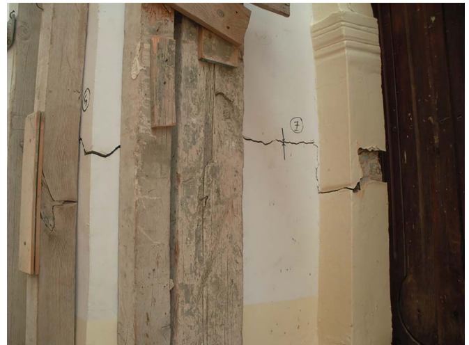
Fig. 2. Al-Mushat mosque, monitoring cracks on a wall.
