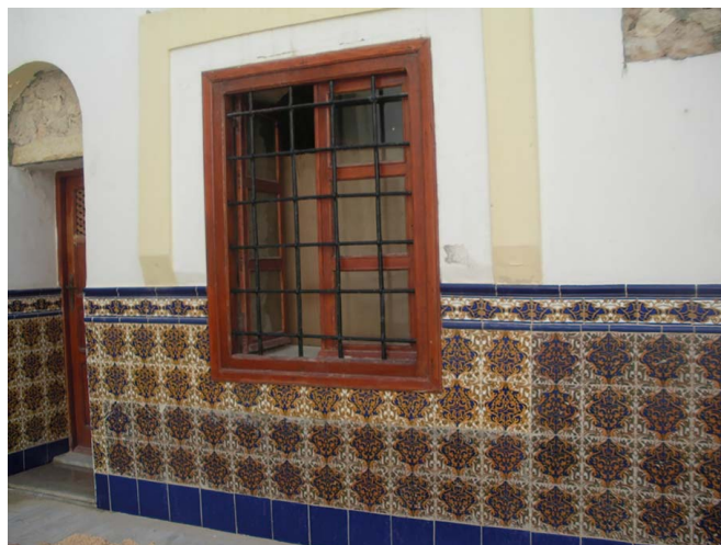
Fig. 18. The former French consulate, distinguishing old and new ceramic tiles.
