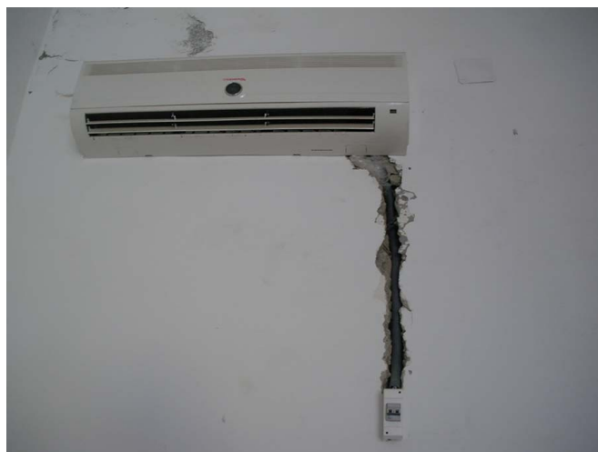
Fig. 19. The former French consulate, electric wires were lined randomly in walls.
