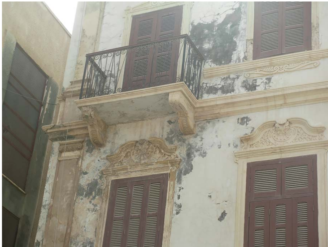
Fig. 11. The former bank of Rome, high dampness in walls.
