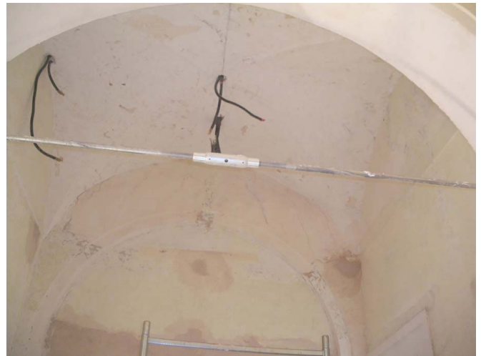
Fig. 7. The Islamic museum, prestressed metallic ties were used to support arches.
