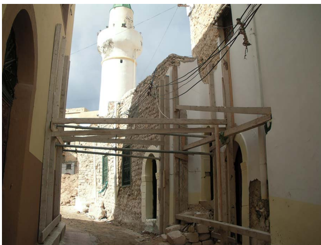
Fig. 1. Al-Mushat mosque, consolidation of cracked walls during refurbishment work.
