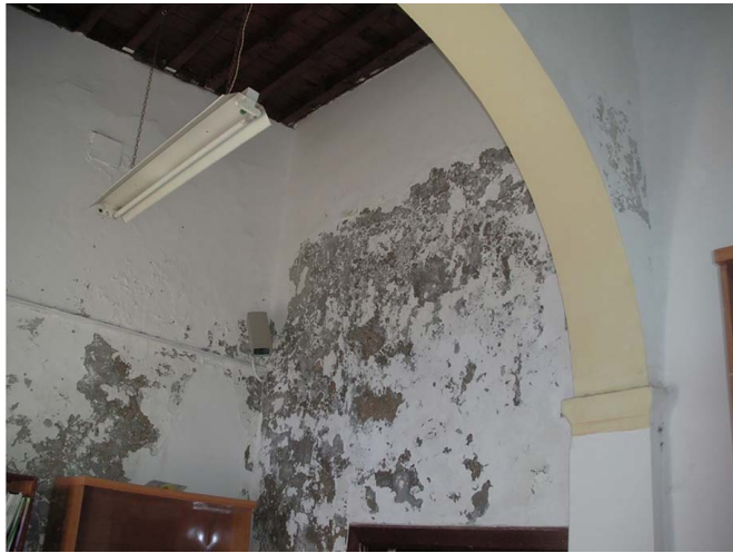
Fig. 10. The former British consulate, dampness in walls.
