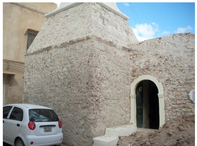
Fig. 8. Al-Mushat mosque, repair work depended on removing all plastering layers.
