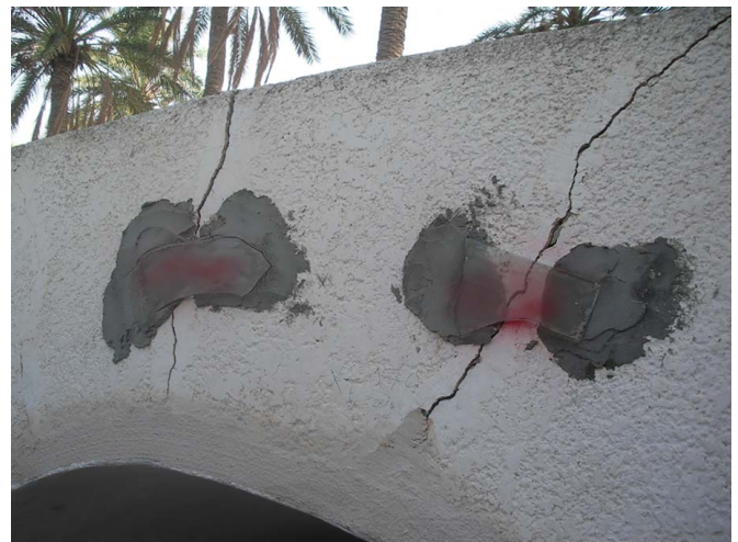
Fig. 3. The Islamic museum, checking the expansion of cracks.
