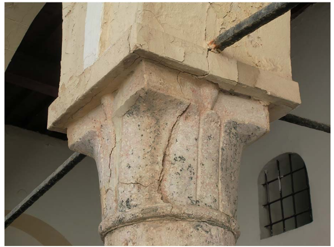
Fig. 6. The former British consulate, inappropriate metallic ties were used to support arches.
