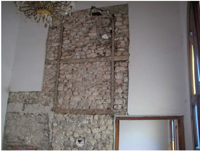
Fig. 9. The former French consulate, removing old plaster layers of the affected areas.
