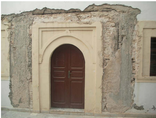
Fig. 5. The former British consulate, exaggerated and inappropriate use of reinforced concrete.
