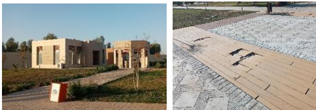
Fig. 4: Pathways' Pavement at Peshmerga Park A. cement block B. wood plastic flooring
