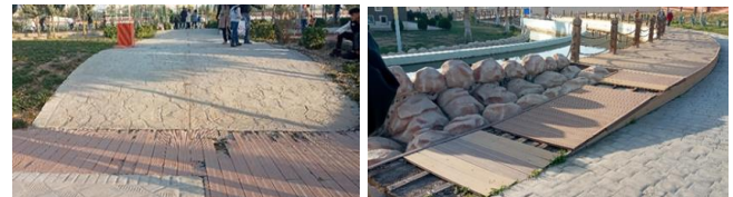
Fig. 5: Ramps at Peshmerga Park A. sloped pathway B. discontinuity of a ramp surface
